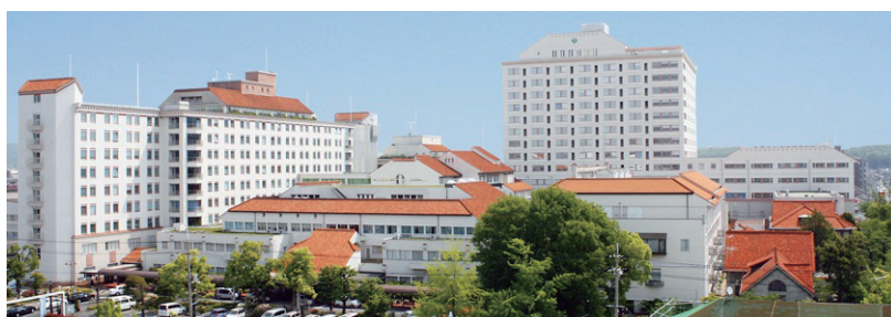
Fig.1 Kurashiki Central Hospital
