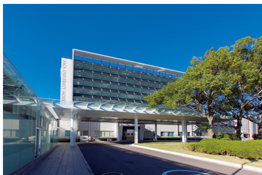
New south clinical service building with helipad
